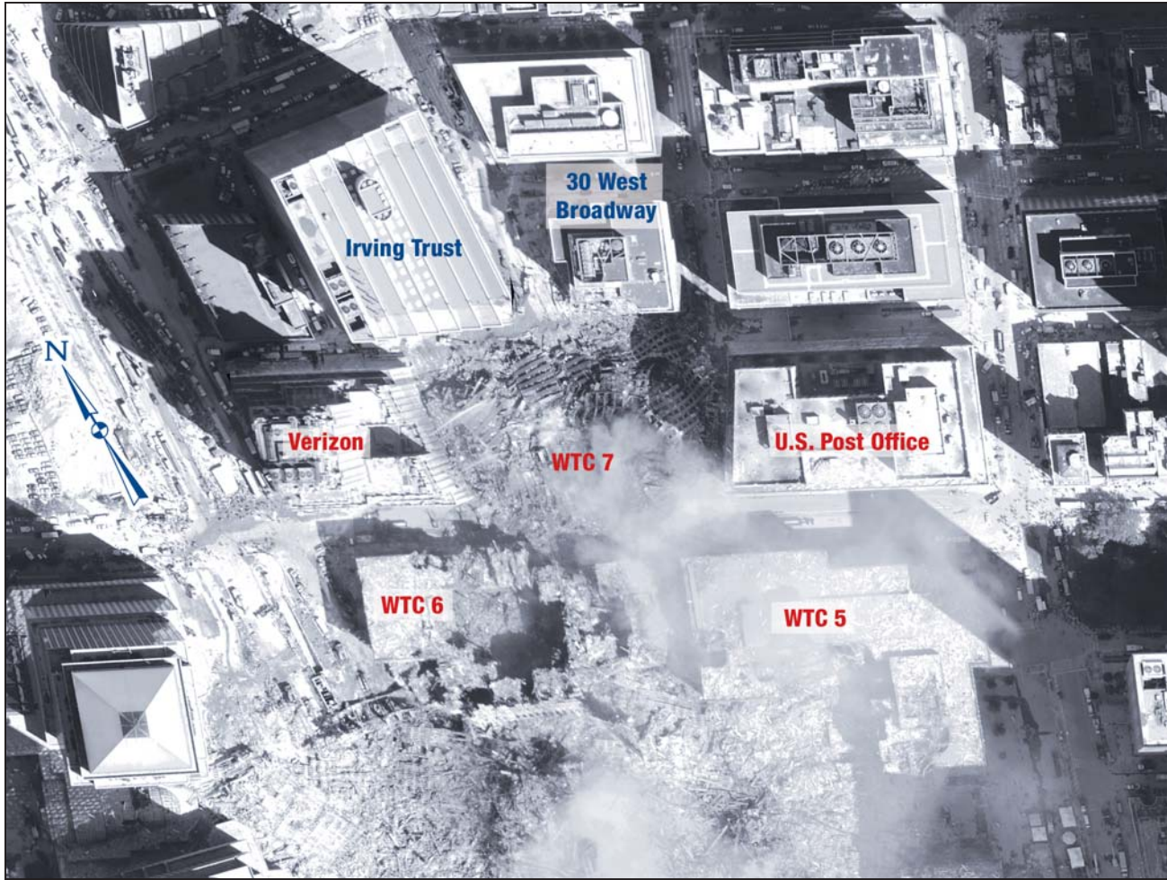
Figure 5-26 Debris generated after collapse of WTC 7.
