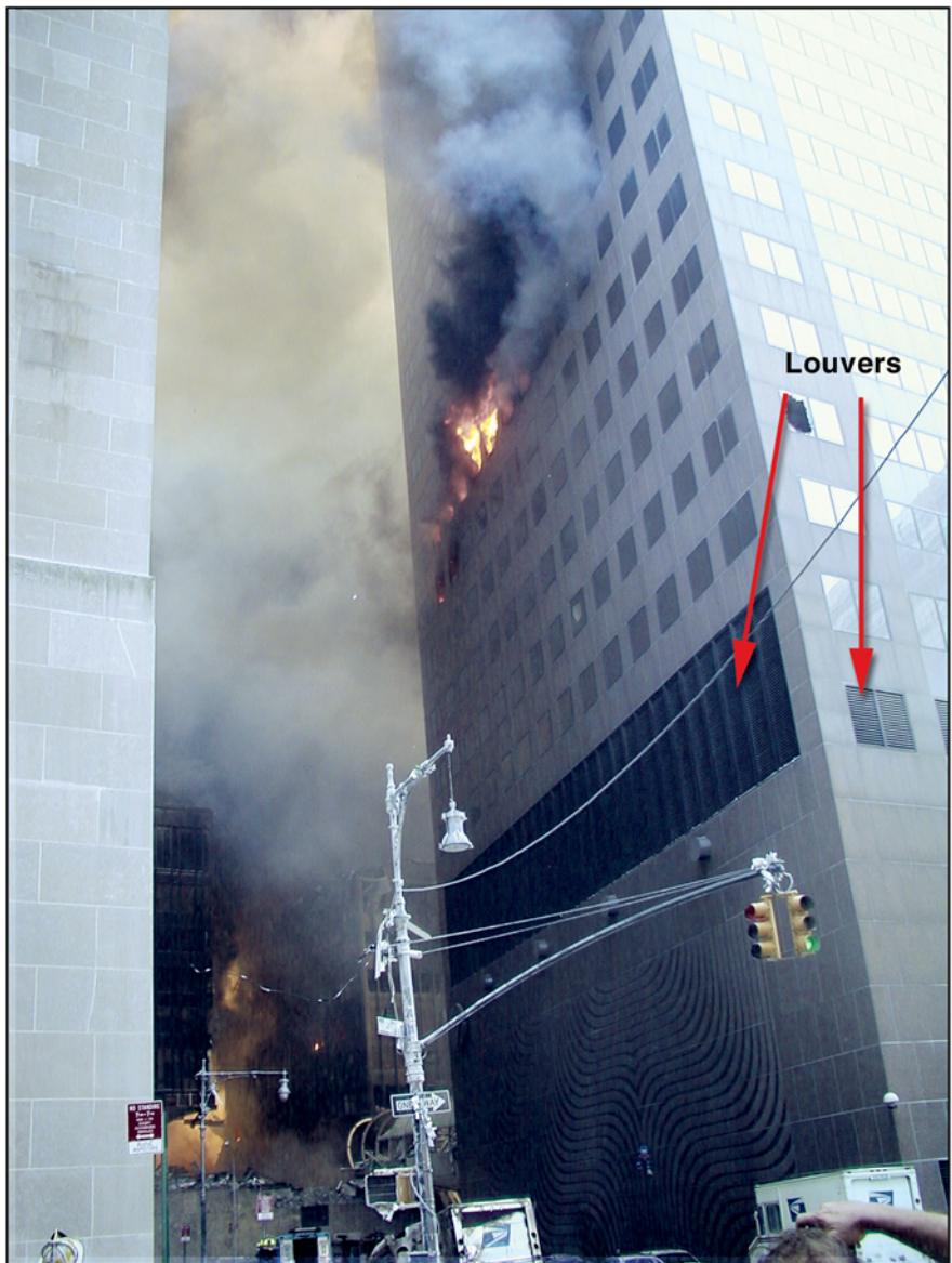
Figure 5-19 Fires on the 11th and 12th floors of the east face of WTC 7.
