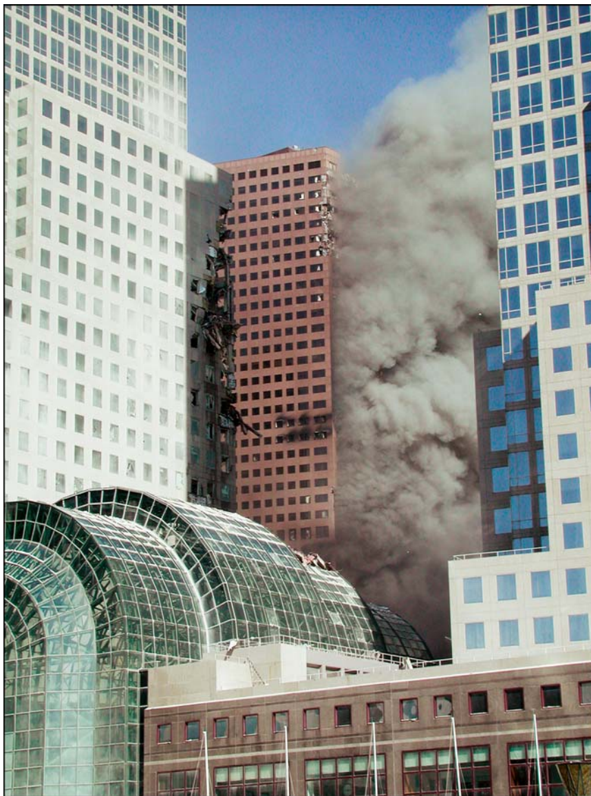
Figure 5-17 Building damage to the southwest corner and smoke plume from south face of WTC 7, looking from the World Financial Plaza. Note damage to WFC 3 in the foreground.
